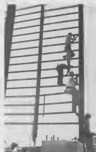
THERE ARE different ways to reach above the normal arm's length. Photo shows Lago workmen climbing a wide ladder.
